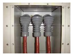
**Silicone Rubber** Straight/right angled **bushing boot** (sealing sleeve)
